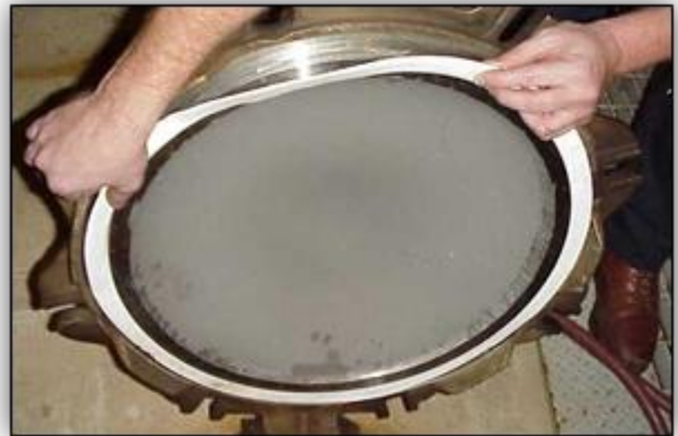
Figure 9: Installation of gasket.
