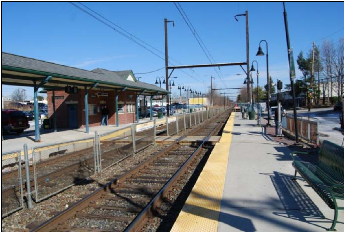
Figure 1: Example of intertrack fencing with crossing surface providing for desired pedestrian movement between passenger platforms.
