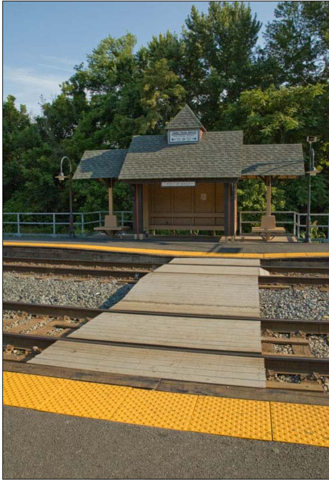
Figure 1: Example of visually contrasting surface materials used at a pedestrian crossing.
