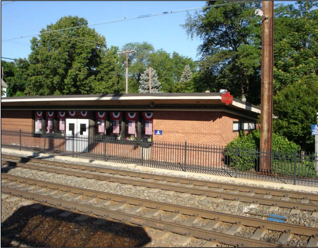
Figure 13: Example of platform edge fencing.
