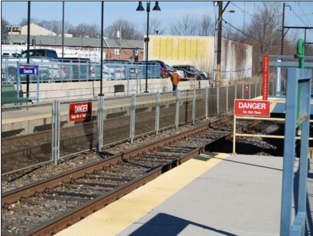
Figure 12: Example of station signing clearly indicating areas from which pedestrians are prohibited.
