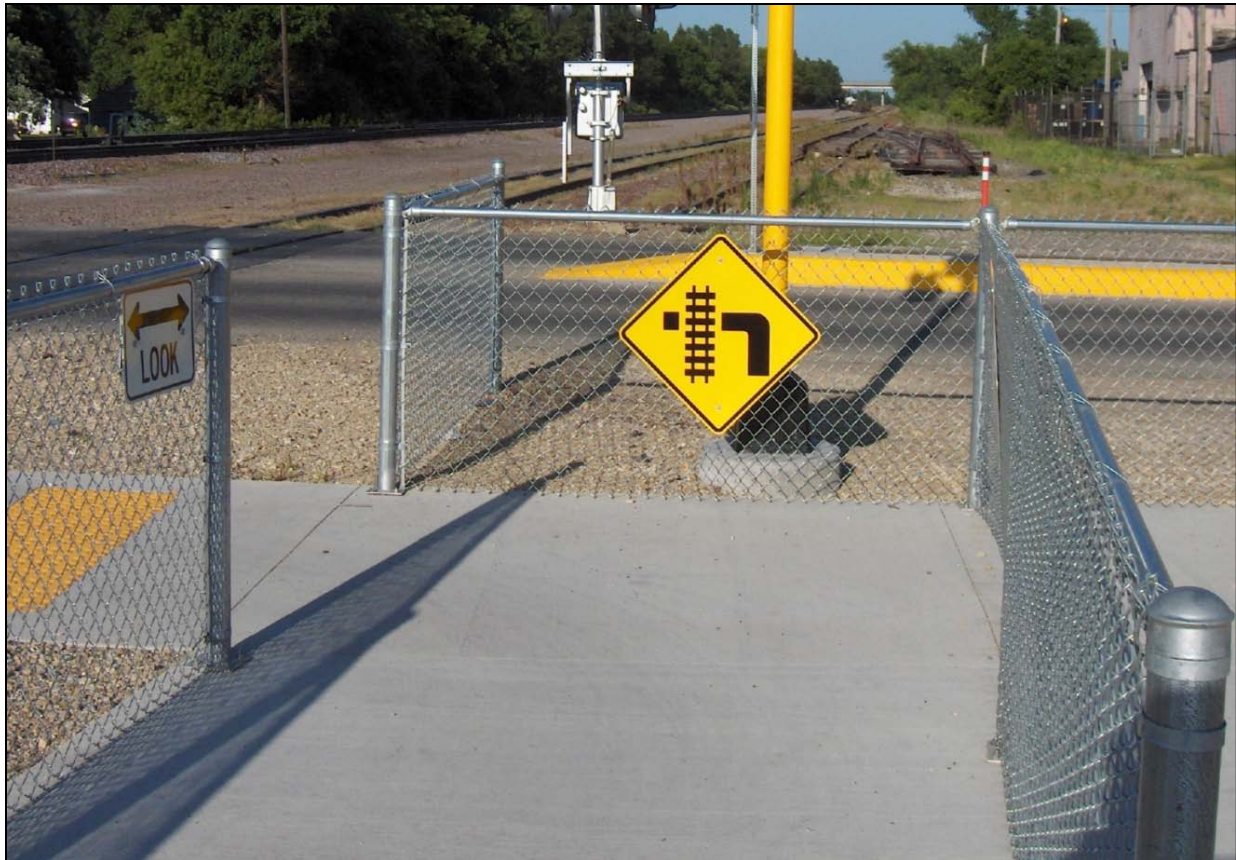
Figure 6: Example of a warning sign combined with right-of-way fencing to channelize pedestrians to the desired crossing location.
