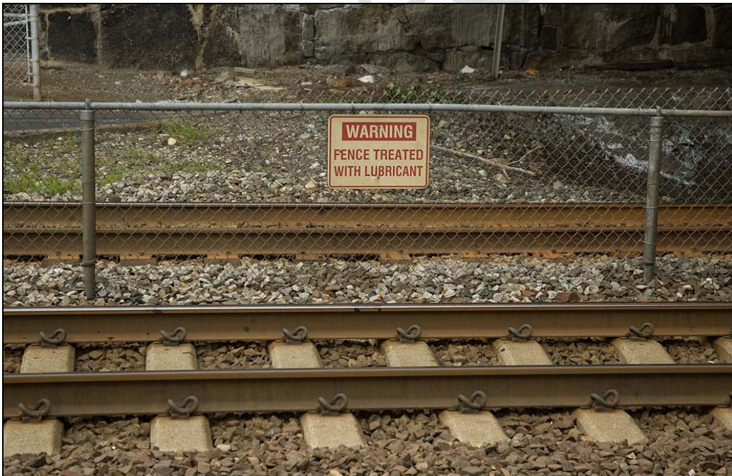
Figure 14: Example of signing and strategy to reduce “fence-jumping” by regular commuters who stubbornly insist on using a favorite shortcut.
