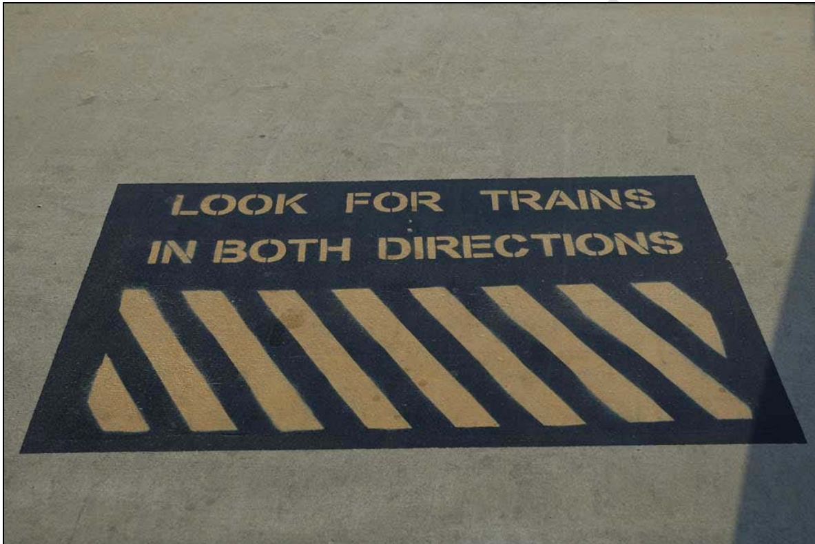
Figure 9: Example of a clear, concise warning message communicated by this pavement marking.
