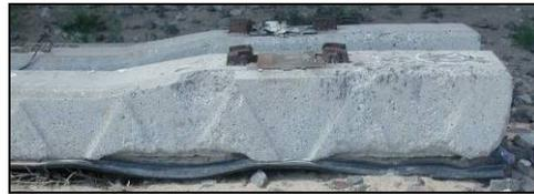
Figure 16. Concrete Ties with Cast-In Rubber Pads.
