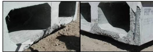
Figure 2. Damaged Concrete Box Girder A (left) before Repair. Figure 3. Damaged Concrete Box Girder B (right) before Repair.
