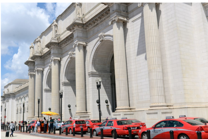
Cabs at Washington Union Station, the southern terminus of the NEC
