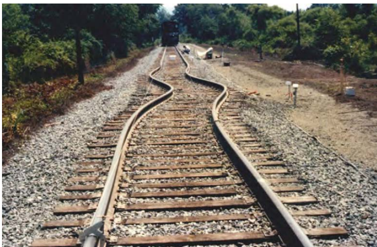
Figure 7.15-7: Example of Rail Buckle from Extreme Heat
