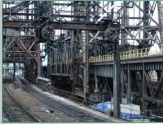
NEC Rail Network: Aging infrastructure, limited track capacity, critical chokepoints.
