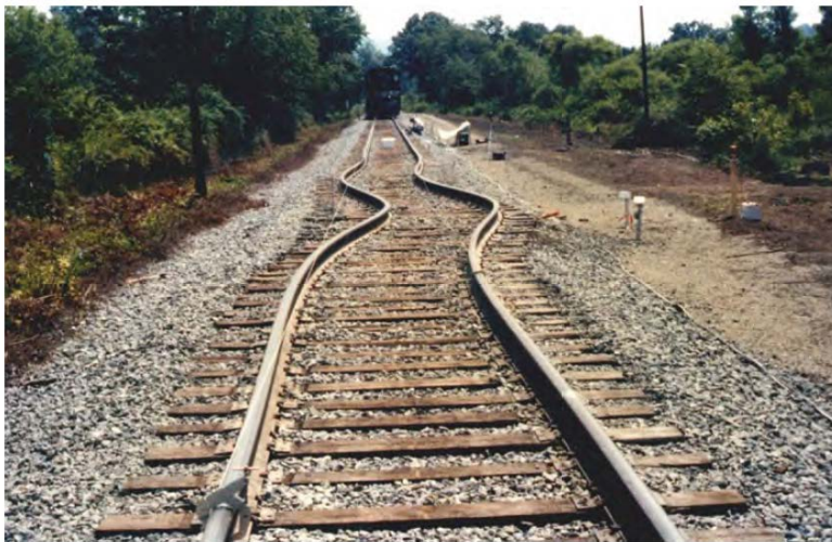
Figure 7.15-17: Example of Rail Buckle from Extreme Heat
