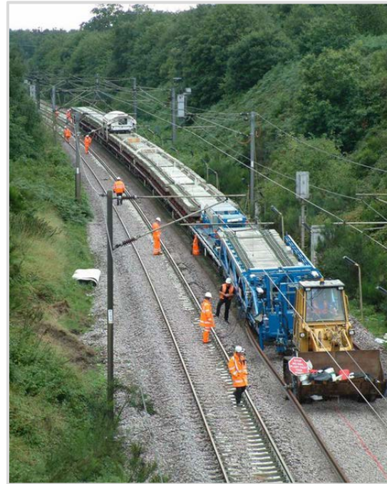
Figure 8-4: Typical New Track Construction Machine
