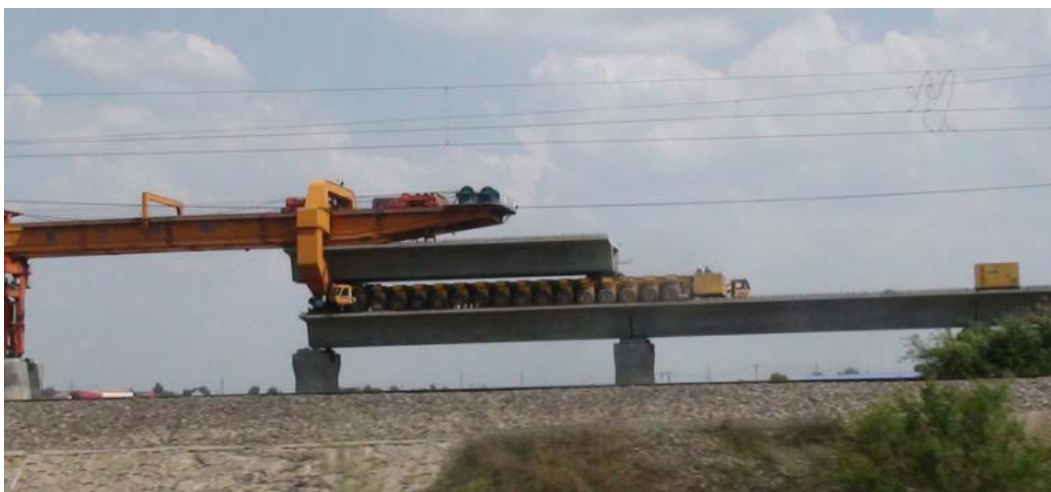
Figure 8-3: Gantry Crane System for Aerial Structure or Major Bridge Construction
