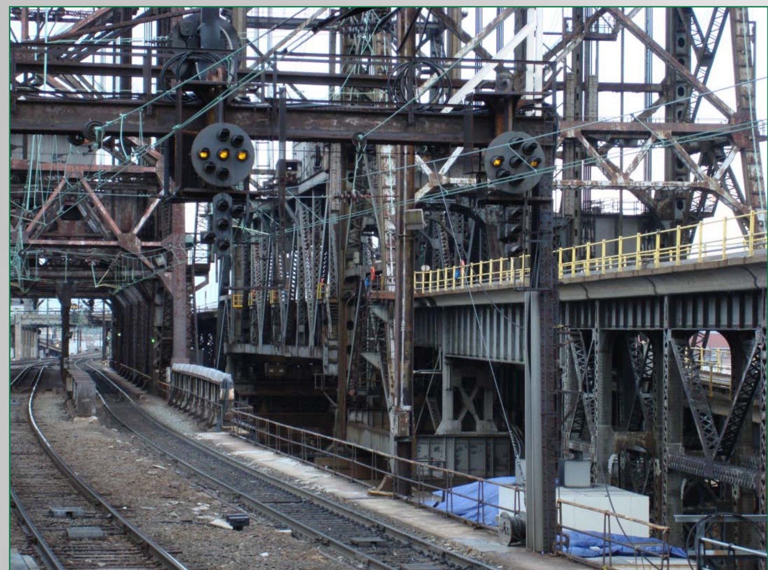
NEC Rail Network: Aging infrastructure, limited track capacity, critical chokepoints.
